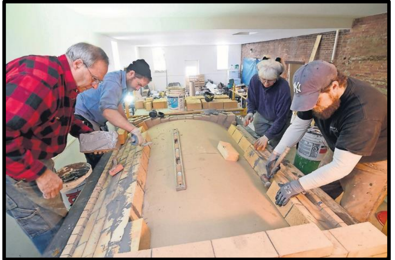
Restoration of the wood-fired oven in the historic Rise Up Bakery adjacent to the Old Labor Hall in Barre
